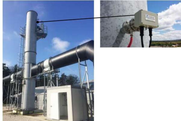
Laser extractive H<sub>2</sub>S ppb continuous monitoring
