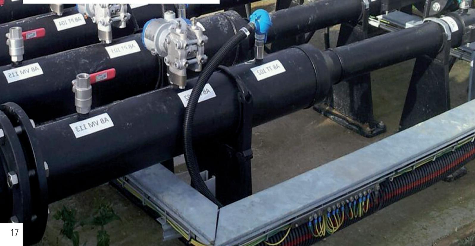
Flow measurement by differential pressure device (orifice plate) for application on gas, liquid and steam.
